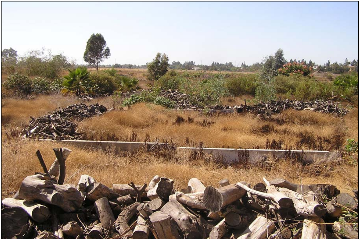
Photograph 22. Overview of the concrete foundation from Site 001, facing west.
