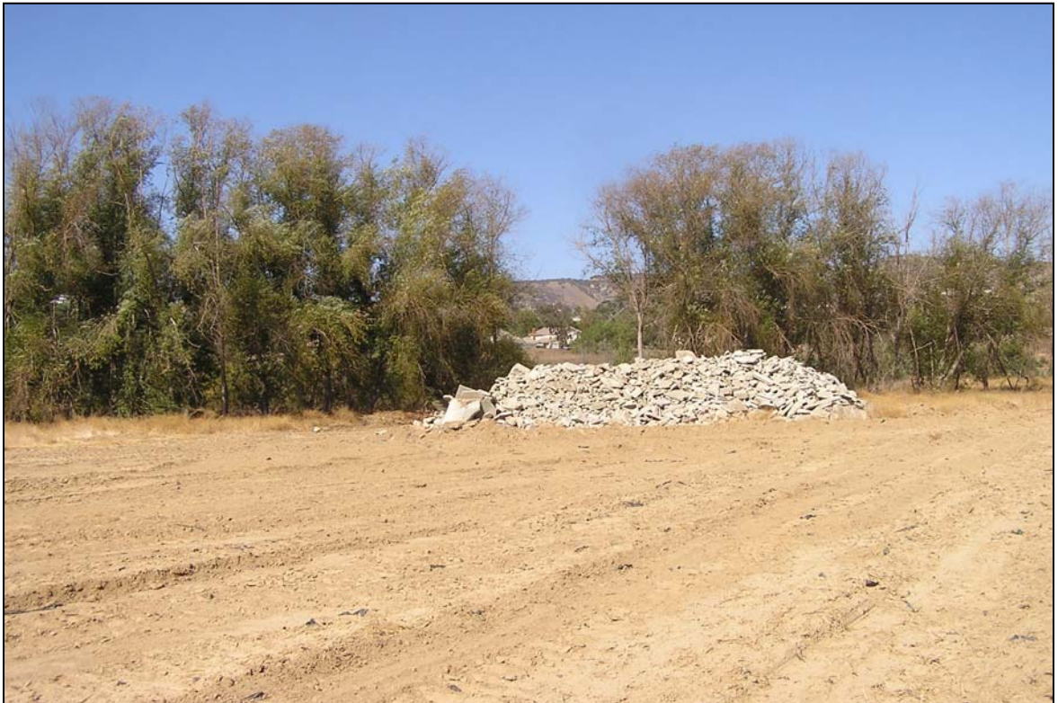
Photograph 16. Overview of the central portion of the project area. This concrete debris pile is also observable on the right side of Photograph 15. View to the northeast.
