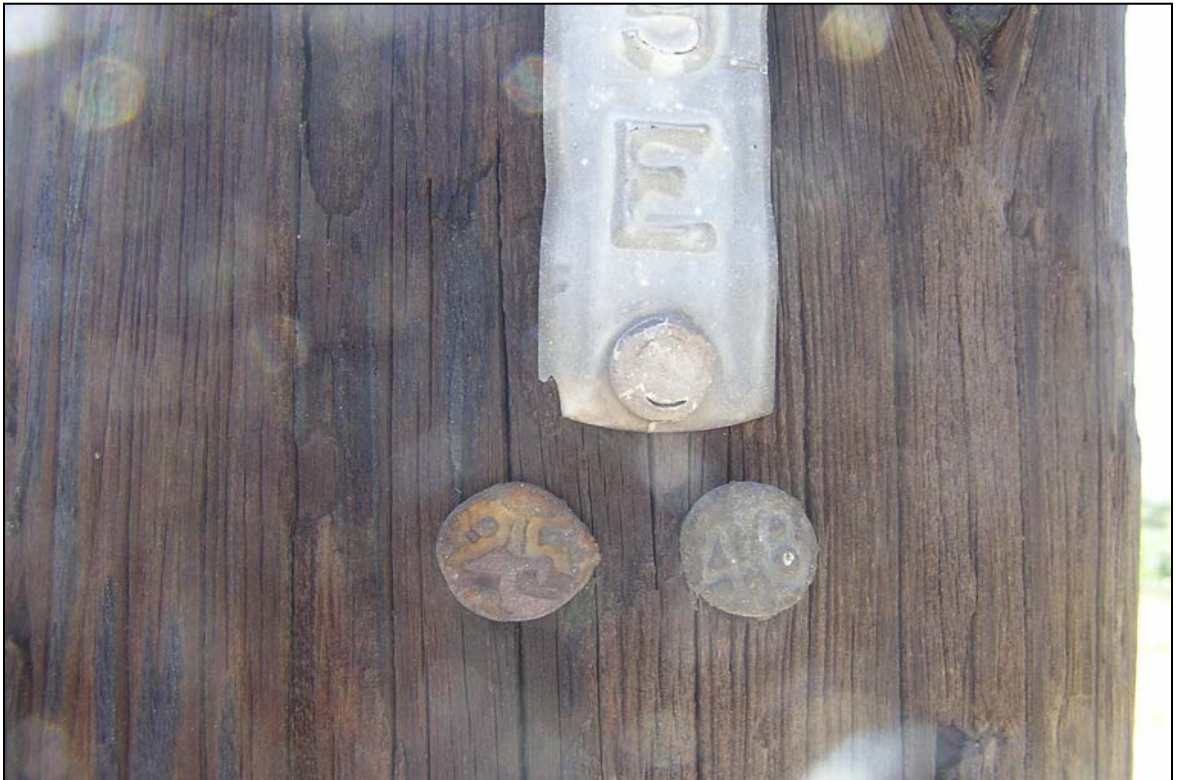
Photograph 24. Close-up of the height and date nails in utility pole 718839E. This utility pole is found to the southeast of the concrete foundation in Photograph 22 and to the west of the lot depicted in Photograph 23.
