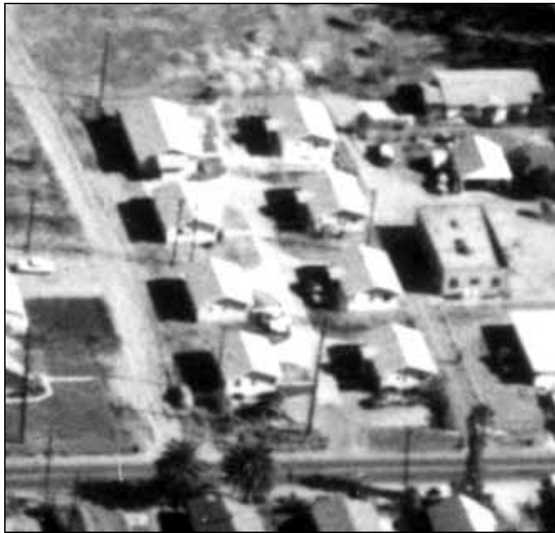
Figure 24: Bungalow court on Hewes Street at Philo Avenue, view east, November 17, 1962 (UCLA Air Photo Archives).
