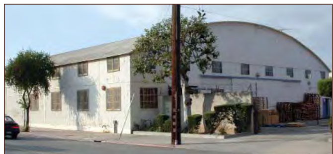
Example of arched roof exterior.
