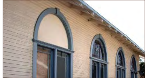
One of the arched leaded glass windows of this church building has been partially enclosed. Rehabilitation should include the restoration of the original window.
