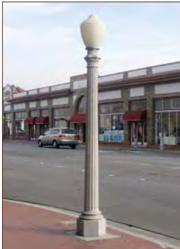
Pedestrian-scaled acorn-globed concrete light fixture.
