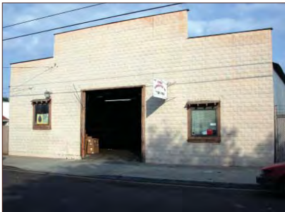
The distinctive pressed tin front of this industrial warehouse building is a rare example.
