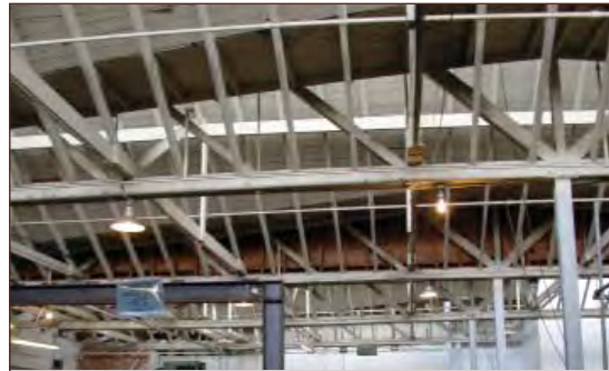
The complex roof truss system in this packing house building not only provides structural support, but is a significant feature to retain during rehabilitation.
