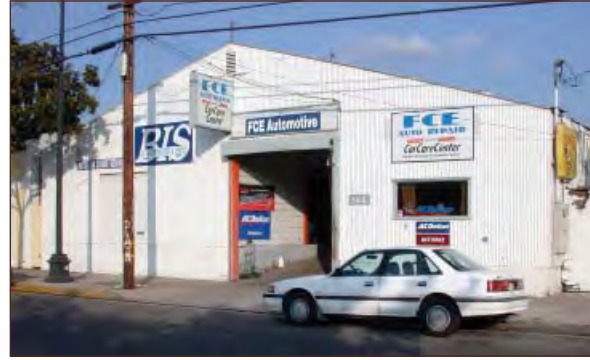
Auto-related building clad in corrugated metal.
