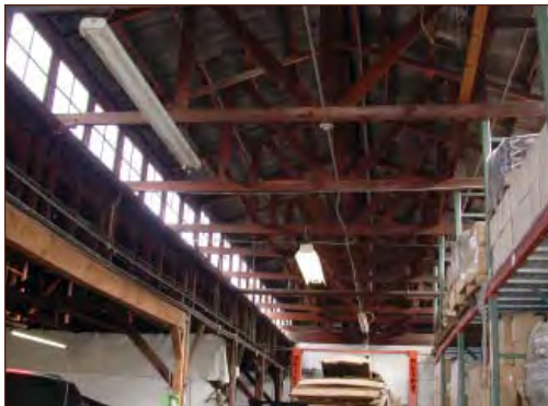
Example of clerestory windows and monitor roof.
