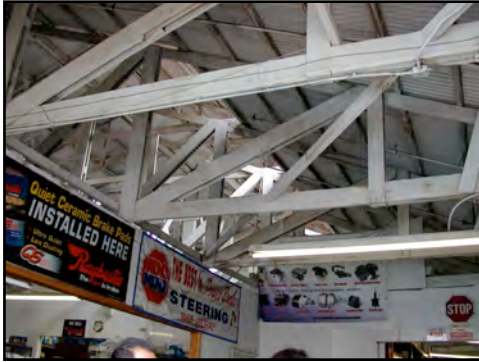
Left: interior showing truss roof system; right: front (eastern) elevation [14 November 2006]
