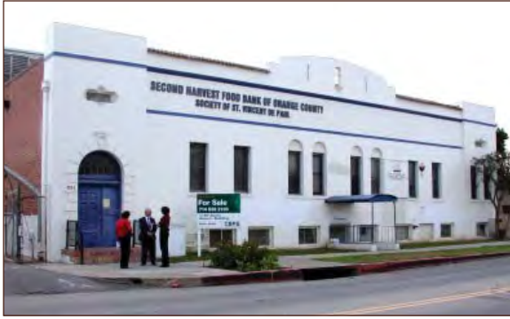
Packing house constructed of brick and stucco-clad.
