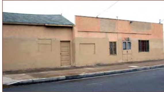
These non-contributing buildings may be able to become district contributors if original openings were restored and add-on materials removed.
