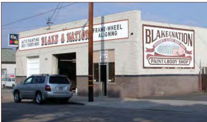
Retain the industrial character of garage bay doors and large windows.
