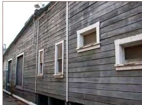
This is a scarce example of original wood siding on this packing house.
