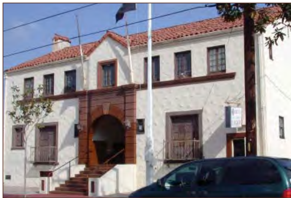
The decorative architectural features of this lodge building are characterized by its prominent raised arched entrance, wrought iron balconies and unusual patterned stucco treatment.
