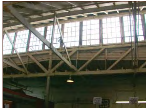
Example of saw-tooth roof interior windows.
