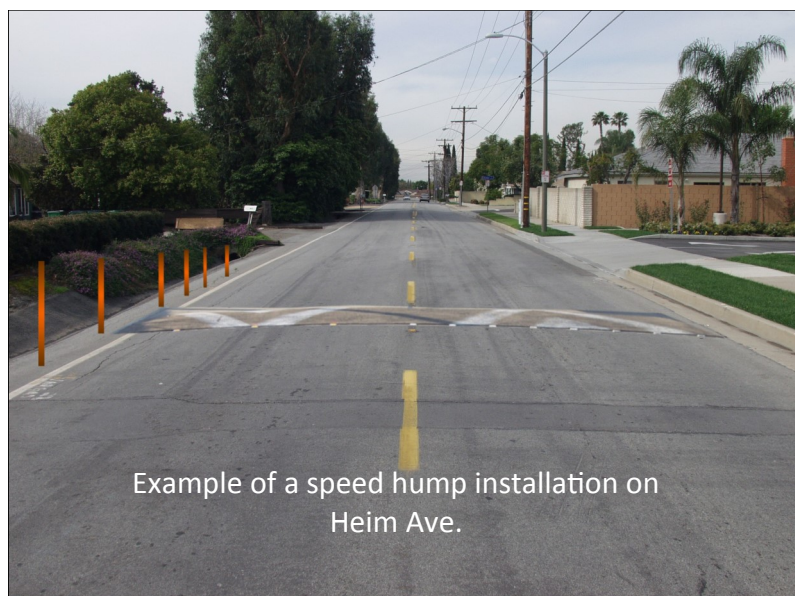
Typical speed hump & warning sign installation
