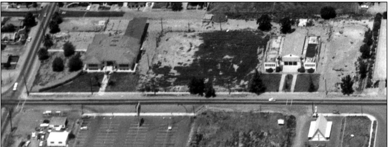
Figure 26: Aerial view of Lincoln Elementary (left, formerly Mexican) and Roosevelt Elementary (right, formerly Anglo) schools on Chapman Avenue at Hewes Street (left), May 17, 1965 (UCLA Air Photo Archives).
