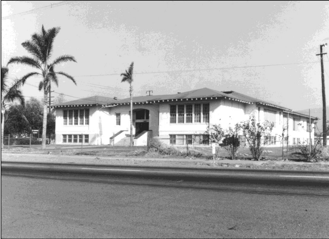
Figure 21: Lincoln Elementary School, constructed in 1913, view northwest, 1950 (First American Title Insurance Company Archives).
