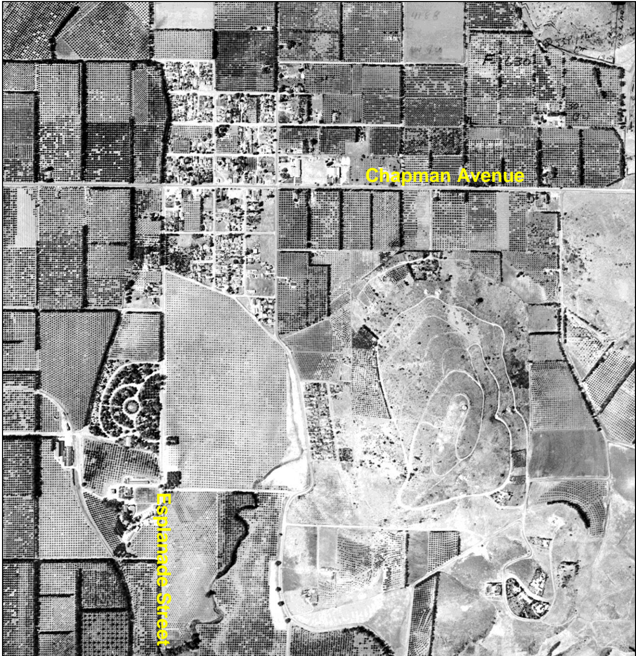
Figure 2: Aerial view of El Modena, 1938. Note Hewes Park at middle left, Chapman Avenue running east-west at middle-top (Orange County Archives).
