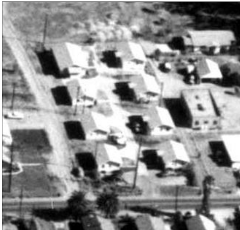
Figure 24: Bungalow court on Hewes Street at Philo Avenue, view east, November 17, 1962 (UCLA Air Photo Archives).
