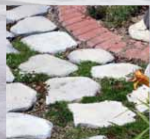
Permeable pavement allows water runoff to infiltrate through the soil and prevents most pollutants from reaching the storm drain system.
