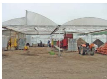
Example of a potting area lacking any type of soil stabilization resulting in significant erosion during storm events.
