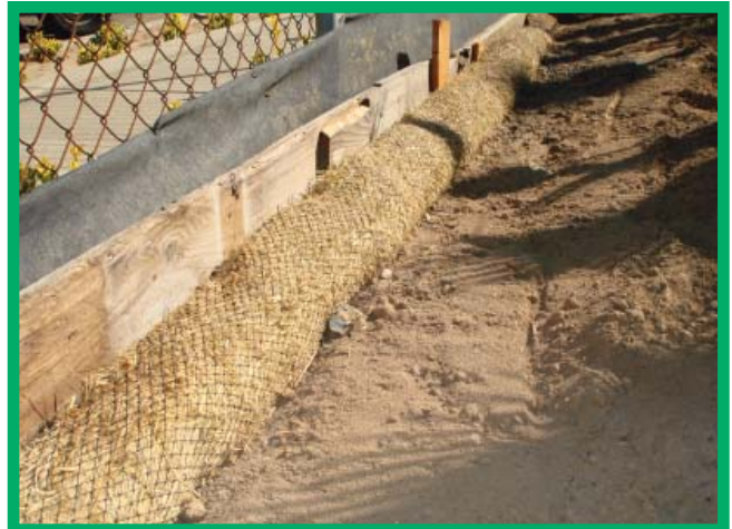
Protect the perimeter of nursery from erosion using wattles.
