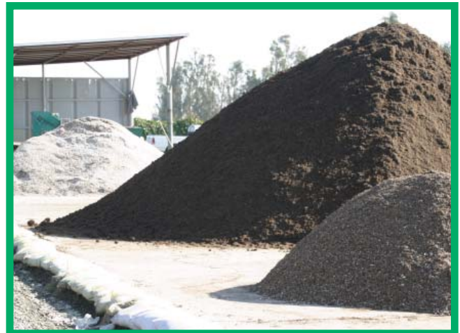
Example of a type of berm (sandbags) around soil piles.
