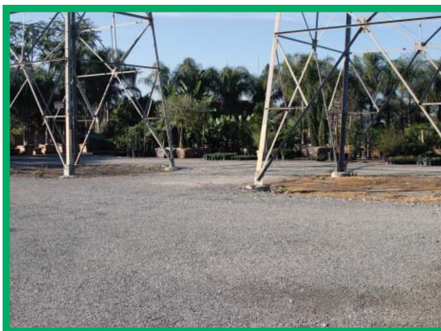
Example of road and exposed access area covered with gravel.
