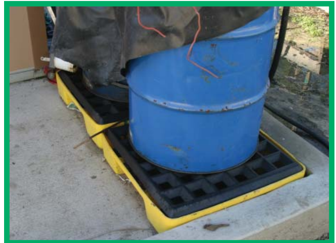
Example of proper storage of chemicals or waste containers in secondary containment areas.
