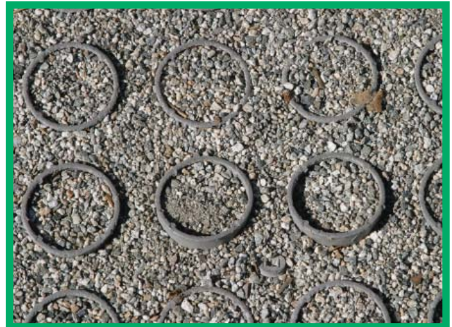
Example of plastic grids used to hold gravel applied to driveway entrance.
