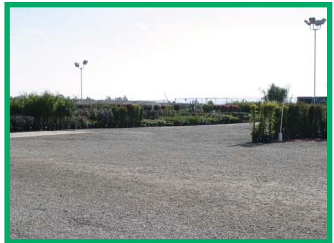
Example of a loading dock protected with a thick layer of 3/4" or larger gravel.
