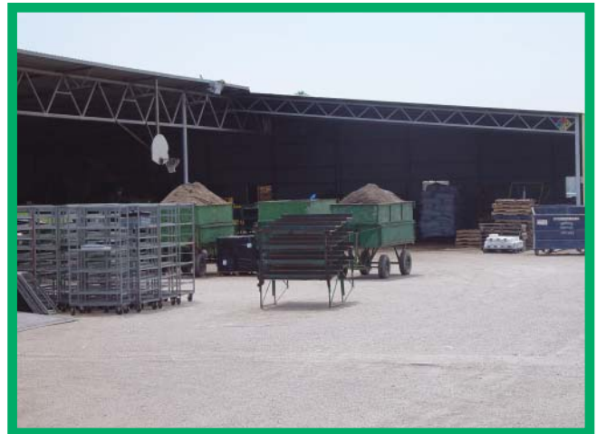
Example of a permanent structure covering a potting area reducing the exposure of loose soil from storm events.
