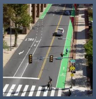
Class II - Standard Bike Lanes (Class II) are lanes for bicyclists adjacent to the outer vehicle travel lanes. These lanes have special lane markings, pavement legends, and signage. Bicycle lanes are generally five (5) feet wide. Bike lanes can be enhanced with green paint or a buffer. Adjacent vehicle parking and vehicle/pedestrian cross-flow are permitted.
