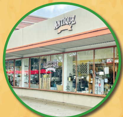
K ALPHA BETA MARKET Constructed in 1949, the Alpha Beta Market was a "modern" addition to the Plaza, responding to the city's growing population after World War II.
