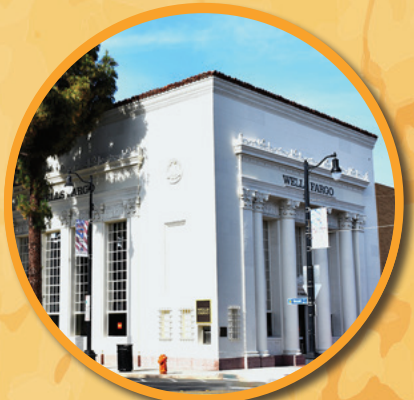
C 101 E. CHAPMAN AVE. Since 1886, this site has held a bank. The original brick building was constructed for the Bank of Orange. In 1927, the building was demolished and replaced with the Classical Revival building for the First National Bank.
