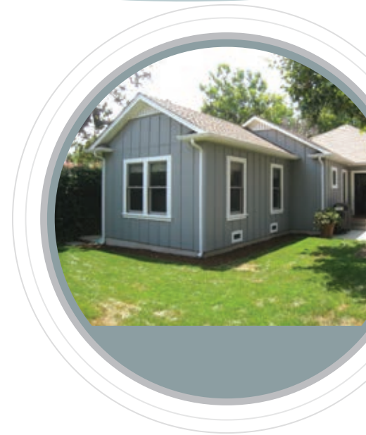
This small rear addition is differentiated from the historic house through the use of board and batten siding which complements the horizontal lap siding on the original building
