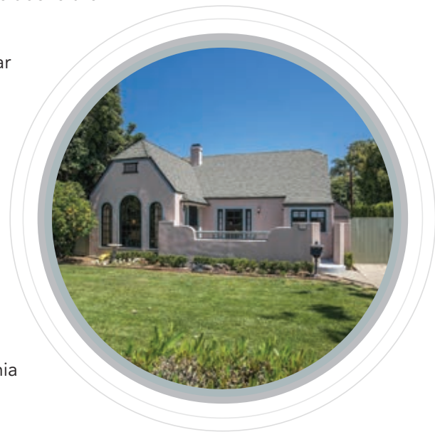
The back side of this roof would be an appropriate place for solar panels
